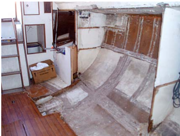
Port side after stripping out the old interior
